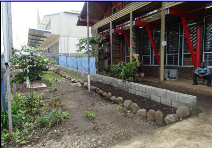
The front of CIC head office in Goroka getting a facelift with an extension of the car park and new fencing, thanks to PPAP
