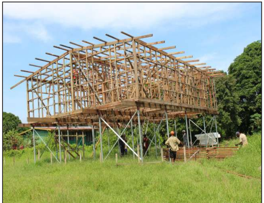
The manager's house currently under construction
