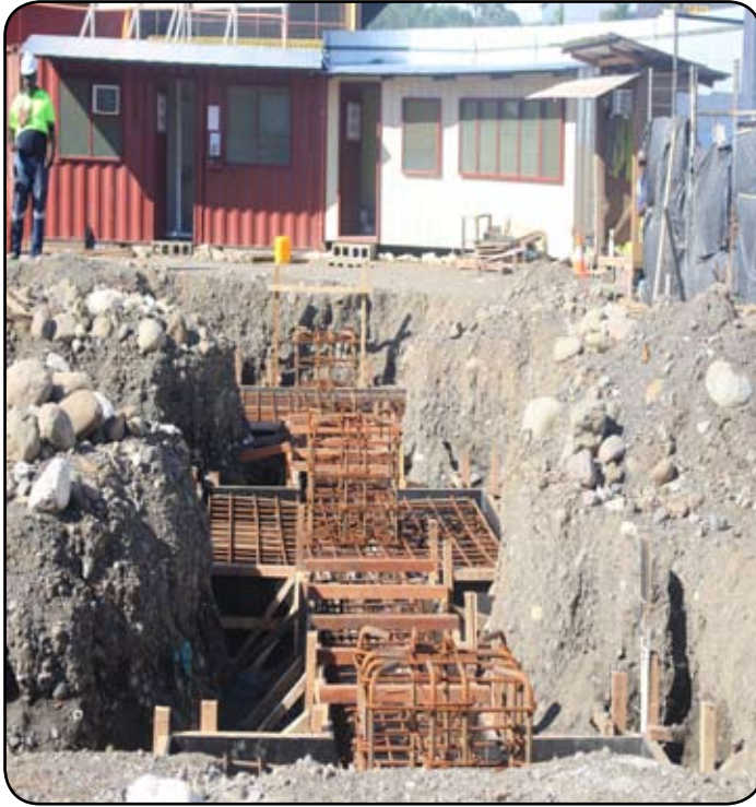
Photos of the Lae Exports Office in the initial construction stage.
